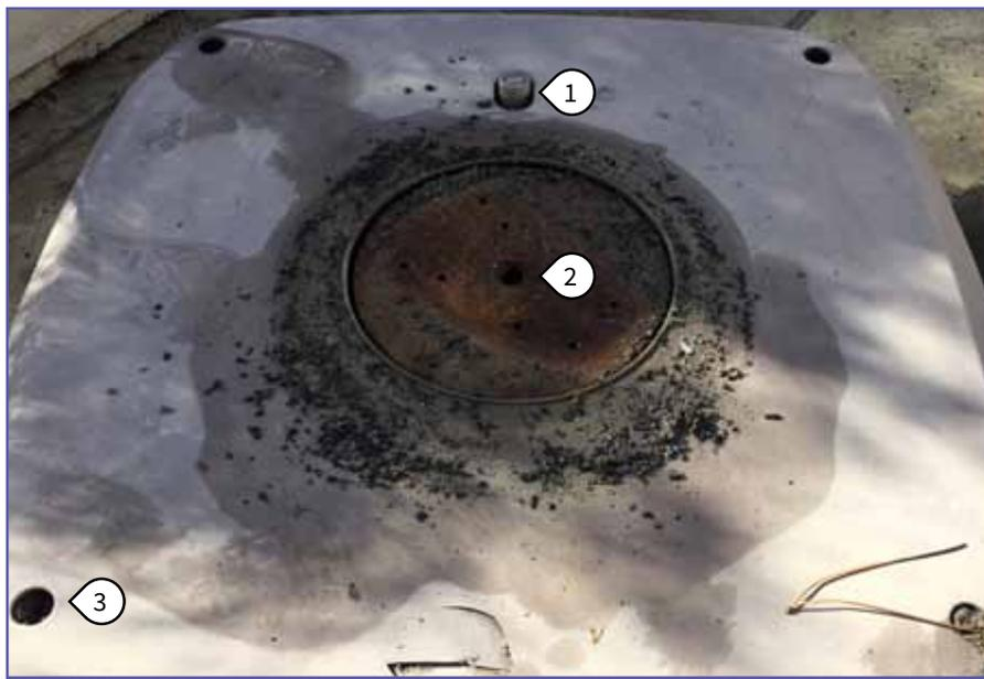
This is an OTU base which has rusted due to sea air (salinity) and a clear indication that it hasn't been maintained correctly.
